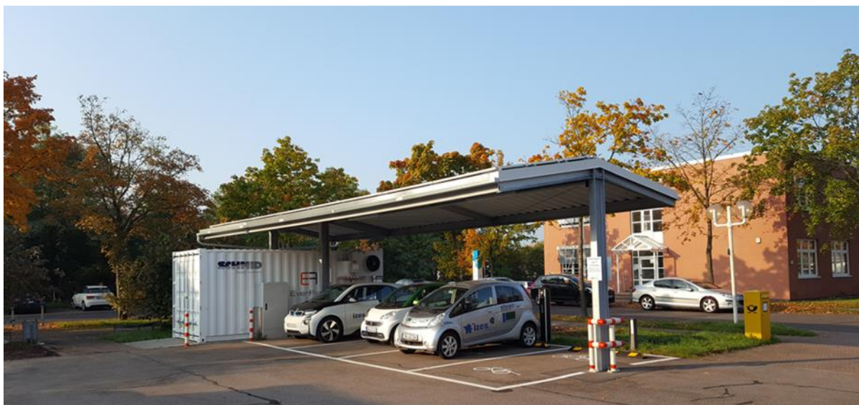
Fig. 3. The IZES solar carport for battery electric vehicles, including a PV array on the roof as well as the containerised Vanadium-Redox-Flow-Battery in the background (Source: IZES)
